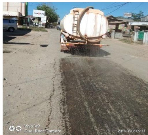
Figure 4. Spraying water in project site.
